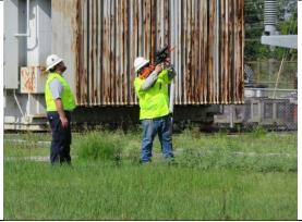
The use of a paint marker with grease balls proved to be effective in reducing forces to manually open a MOAB and close a ground switch. The use of the paint marker allowed lubrication to be conducted from a safe distance. Safety briefing related to the proper and safe use of the paint marker should always be conducted as part of a JSA to ensure safety and accuracy in hitting that targets with the grease balls.
