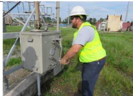
Avoid standing directly in front of the MOAB while turning the switch handle as shown above as this position of operation causes twisting of the trunk and increases the risk of a back strain.
