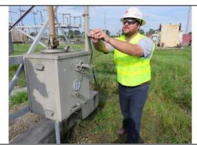
After l;ubrication, opening the MOAB should be conducted standing as shown (on the side of the MOAB). This is the best position to be in to operate the handle as it reduces the amount of trunk twisting and back strain.
